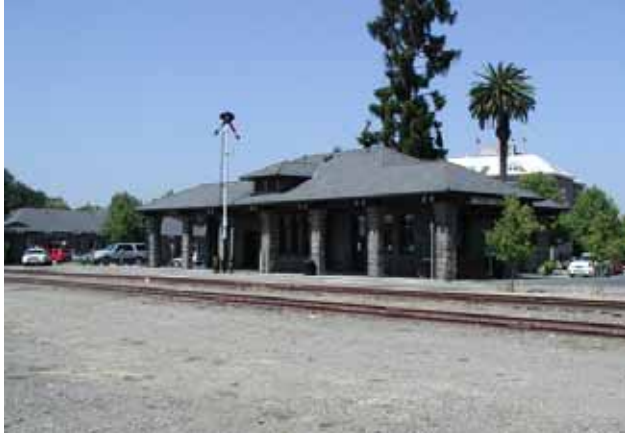
Northwestern Pacific Railroad Depot was constructed of locally quarried stone in 1904 on the site of an earlier two-story wood-frame depot.
